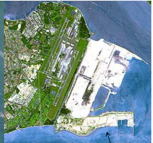
Changi East Land Reclamation Project
